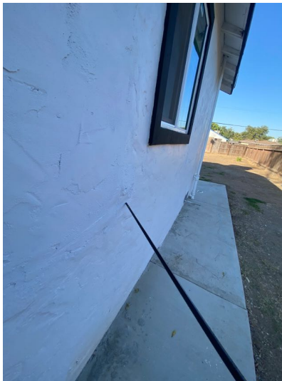
North side of home
