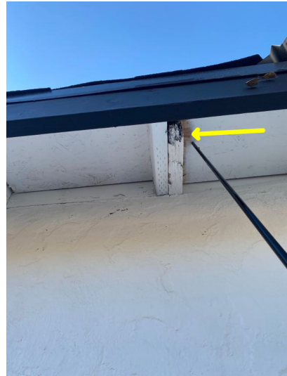
North side of home
