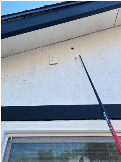
West side of home
