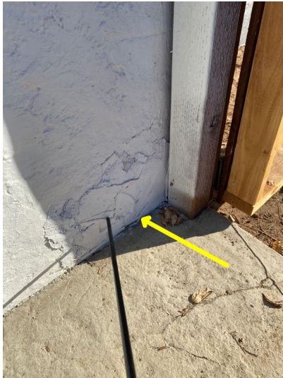
Southeast side of home
