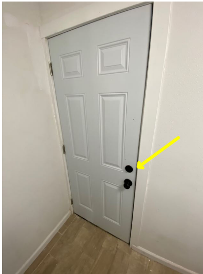
Homes back entrance door
