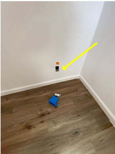
Master bed (east bedroom) west wall
