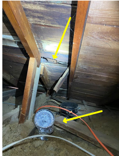
Kitchen exhaust ducting
